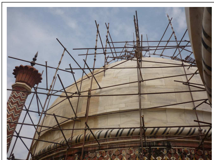
FIGURE 1. A clean surface and an area being prepared for cleaning on a marble Mosque dome at the Taj Mahal
